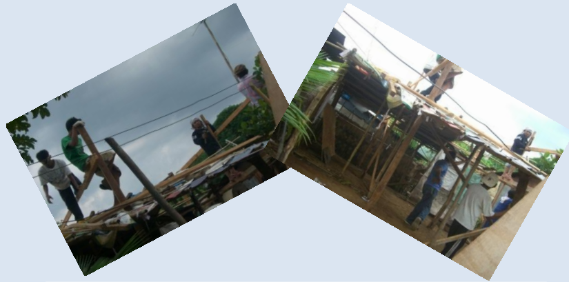
Church people donating labor to work on the house
